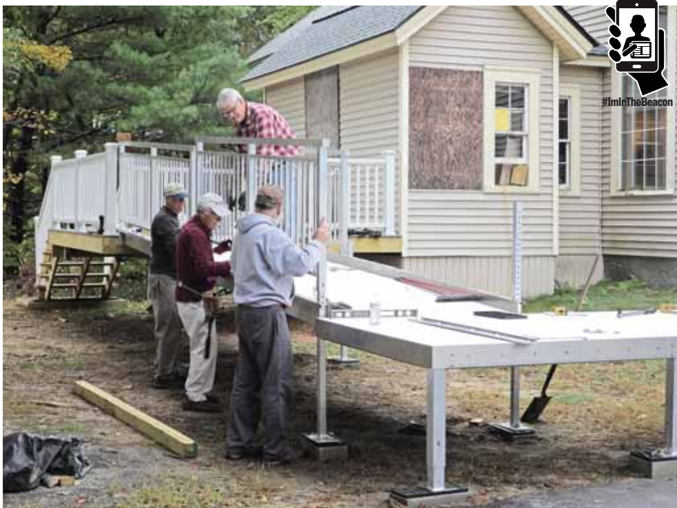
The project to build an access ramp to the Hub building, as part of the Capital Campaign, is underway. Shown at work are Hub volunteers Doug Phelps (on ramp) and Steve Darling, Harvey Pine, and Ken Wells. Photo: Larry Chase
